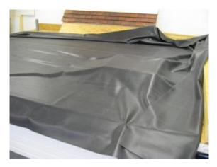
This should be around the 30 minute mark, over which time you will find that the EPDM has settled, and it is in the ideal condition.
