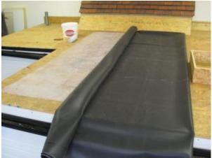
The second is a contact-based adhesive that is stronger and is used to seal down the edges.
