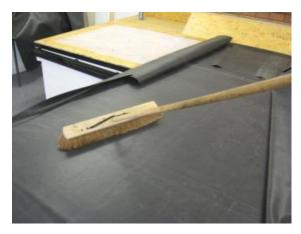
It is important to make sure you firmly adhere the EDPM membrane properly to the roof deck once the adhesive has become tacky.
