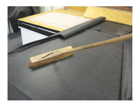
Roll back the other half of the membrane until approximately 100mm of the already applied adhesive is visible and repeat the procedure.
