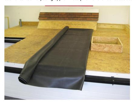
Bonding of the membrane can now begin. Using a 9" roller, apply the water-based bonding adhesive to the timber substrate only.
