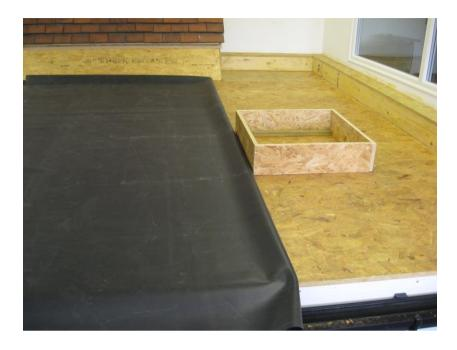
Measure the width and depth of the protrusion and transfer these dimensions onto the folded membrane. Draw an X inside the box.
