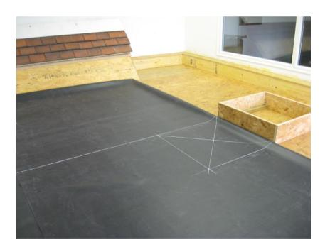
Cut a straight line from the nearest edge of the membrane to one corner, then cut the X mark lines.
