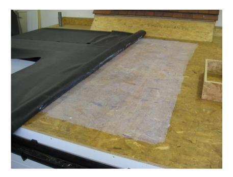
Note that the water-based bonding adhesive does not go right up to the perimeter edge of the roof deck, but instead terminates 100-150mm away. This area is where the Firestone Bonding Adhesive will be applied later. The water-based adhesive can take up to a few hours to grab the membrane completely depending on ambient temperatures, but the use of the Firestone Bonding Adhesive around the perimeter edges secures the sheet in place during this period.
