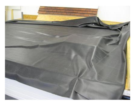
When EPDM membrane is laid in-situ, it can take around 30 minutes to relax. In cold weather conditions, this waiting time will be extended and any folds that are sometimes present in the membrane can take longer to dissipate.
