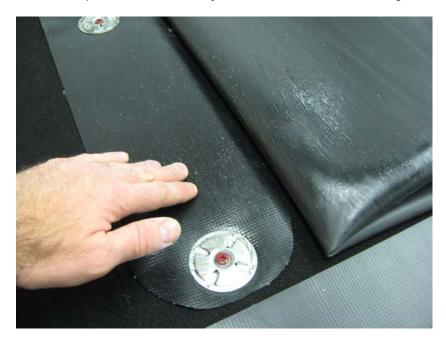
Repeat the procedure on encountering each RUSS strip. Work in one direction e.g. along the width of the roof, then apply the membrane to the strips running down the roof length.
