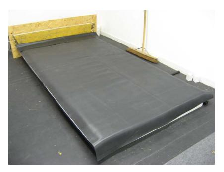
**Please note:** when EPDM membrane is laid in-situ, it can take around 30 minutes to relax. In cold weather conditions, this waiting time will be extended and any folds that are sometimes present in the membrane can take longer to dissipate.
