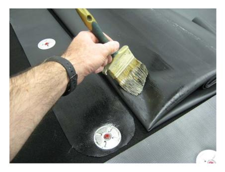
Check the Splice Adhesive is tacky and mate the two surfaces together.
