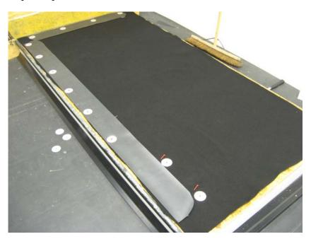
Please note the fixing pattern as shown. The distance between the strips is approximately 1 metre apart, maximum. The higher the wind uplift, the closer the strips need to be. Please ask a member of Permaroof for guidance.
