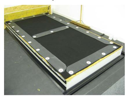
Once the substrate in properly prepared with the RUSS and geotextile undercushion secured, the EPDM membrane can be laid out onto the roof and positioned. Make sure enough membrane overhangs the roof perimeters and upstands, allowing to be trimmed later.
