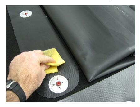
Once the Splice Wash quickly evaporates, Splice Adhesive can then be applied to the same surfaces.
