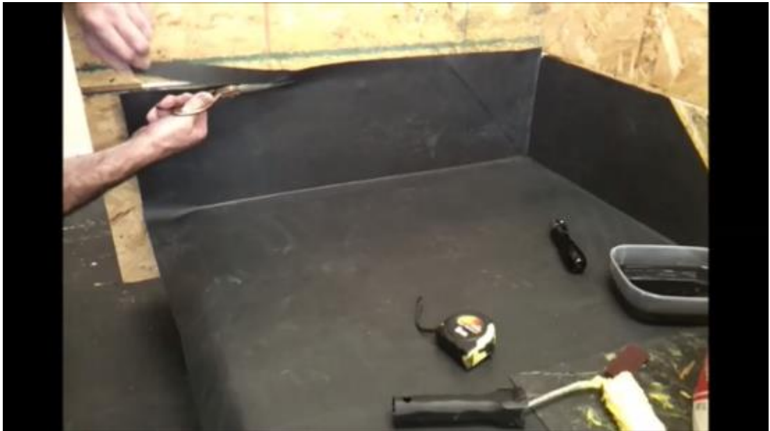
Fig 11: Trimming off the excess membrane.
