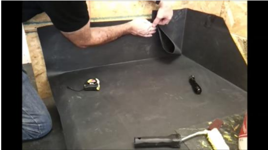
Fig 7: Bringing the two edges together to make the fold.
