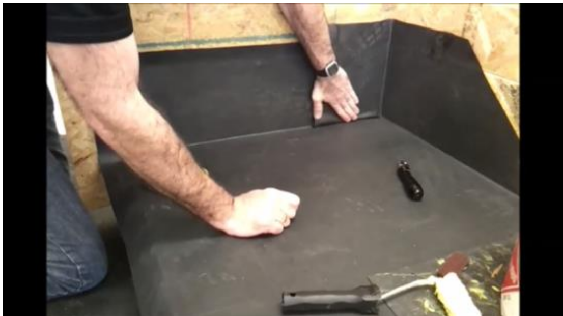
Fig 8: Ensuring the fold is made accurately.
