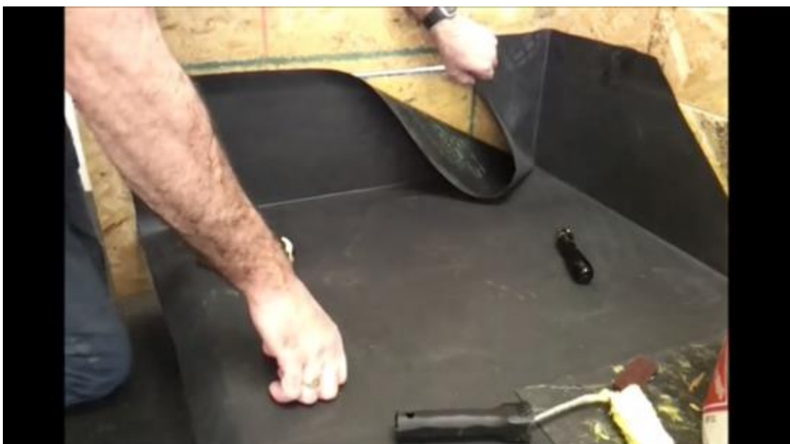
Fig 6: Bringing the membrane over to form the corner.
