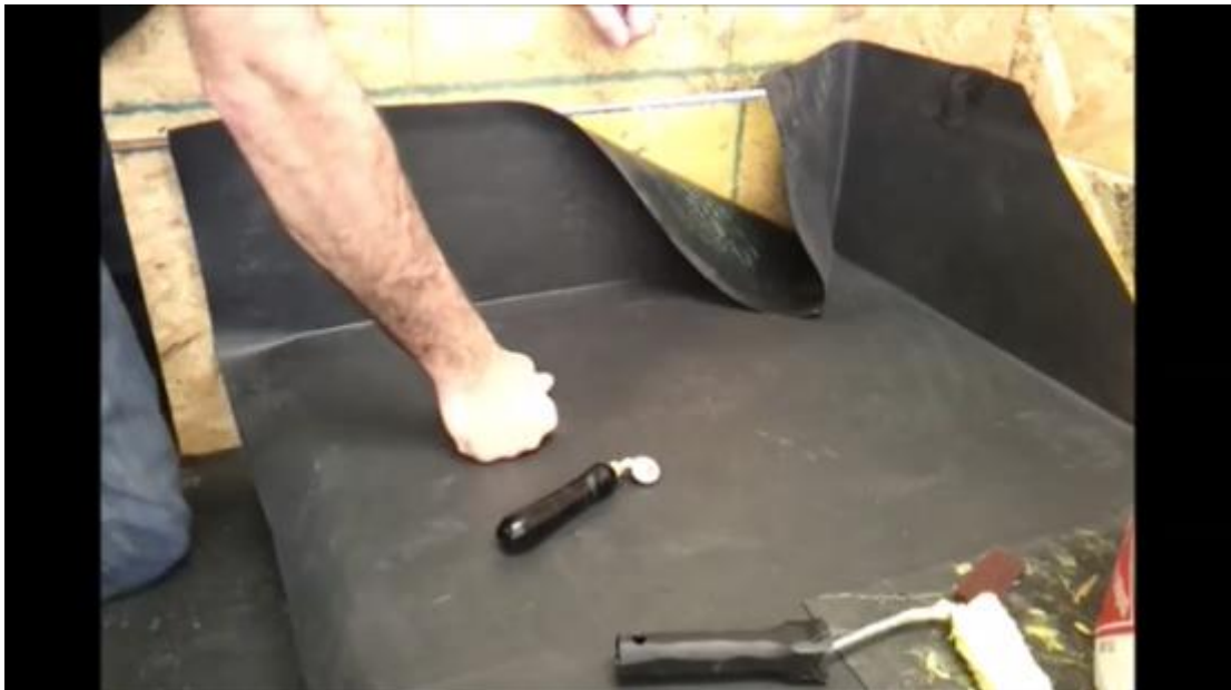
Fig 5: Offering the sheet up to the upstand wall.
