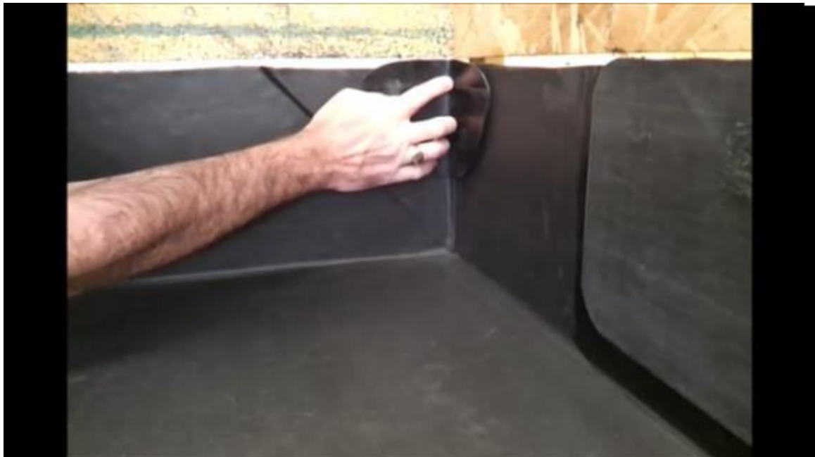
Fig 1: Offering up the FormFlash patch to the internal corner.
