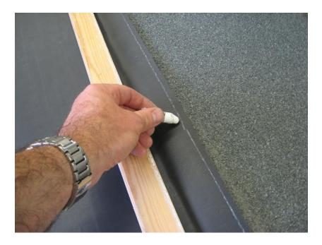
Apply a bead of Firestone Water Block sealant underneath the edge of the membrane.
