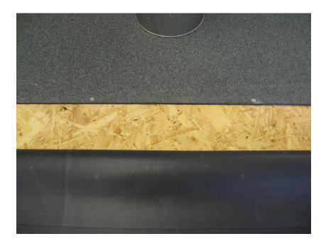
Apply Firestone Bonding Adhesive to the back of the membrane and also the deck...
