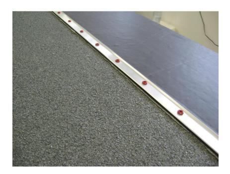
To finish off, apply Quickprime Plus a minimum of 250mm wide centred over the termination bar and running down its entire length. Once tacky, Quickseam Formflash can be applied to this area. Use the rollers to secure the Formflash to the deck.
