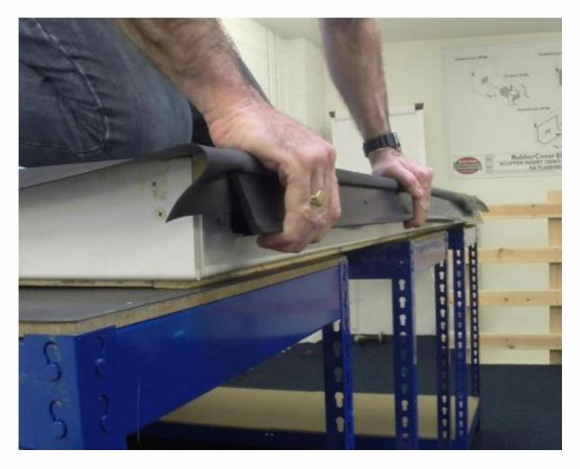
The drip plate can then be attached securely with polytop pins into the pre-drilled holes.
