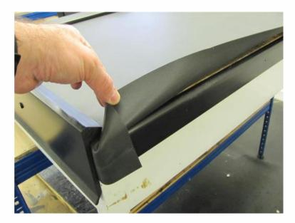
Cut the drip plate to the desired length which will be applied to all existing overhanging roof membrane.
