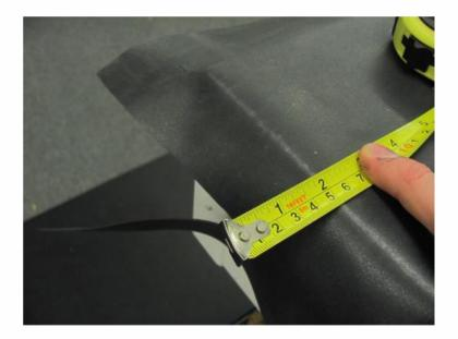
Measure the appropriate length of kerb edge trim needed and cut to size if necessary. Either foam tape or Permaroof Bond and Seal can be used for the watertight seal where it sits on the roof deck. If using foam tape, this seal will only be achieved under compression.
