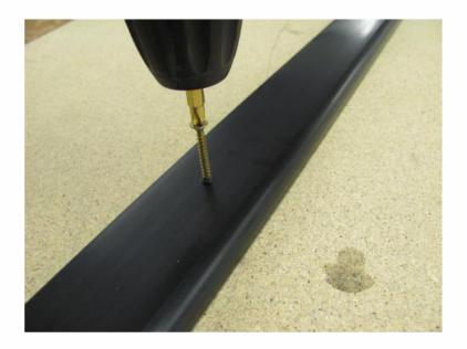
Ensure the top of the backplate is flush with the roof deck surface, then secure.
