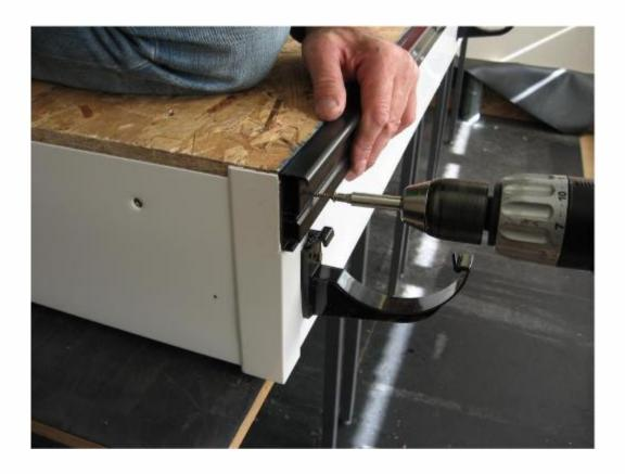
Once the membrane is applied to the roof deck, application of the Permaroof trim system can be completed.
