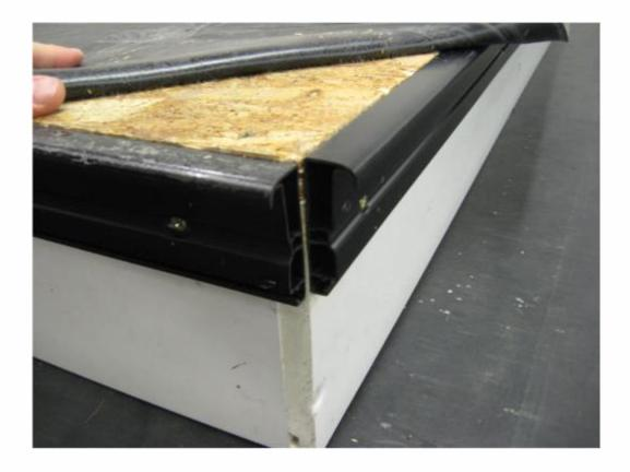
With the membrane hanging over the edges, secure the drip plates.
