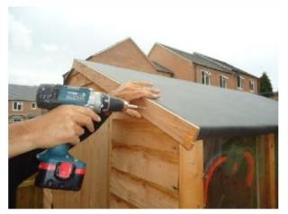
Nail or screw this through the membrane and into the shed timber, ensuring that the nail fixing is below the bead of sealant line to ensure a watertight seal.
