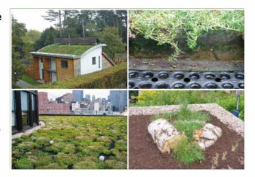
Green roofs consist of several layers of material with a planting medium on the surface. This often assists with creating better insulation for a garden room but needs to have a completely reliable base membrane to ensure a watertight system for the long term.
