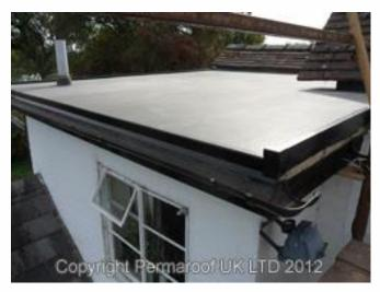
EPDM, when it was first introduced, was commonly used for commercial buildings. This is because it is not only cost-effective, but also because it offered a long-term solution to waterproofing.
