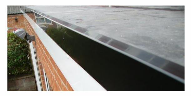
In this guide, we will show you how to install the gutter edge backplate. This is a vital part of the trim system that ensures a watertight seal around your flat roofing installation.
