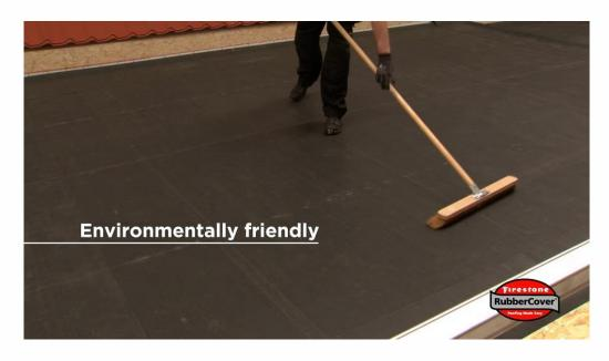
It is important to make sure you firmly adhere the EDPM membrane properly to the roof deck once the adhesive has become tacky. Use a wide-span domestic broom with soft bristles to press down the membrane, the roller to push out any bubbles, and the penny roller into the corners and edges.
