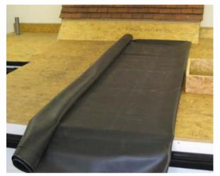
To apply, you need to fold back one half of the membrane, before applying the glue to the roof decking.
