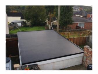
As a rubber roof membrane is typically laid in a single sheet, there are no joins present once the installation is completed. This ensures a comprehensive cover with none of the vulnerabilities that the joins on a felt roof present. If there are rooftop extrusions in the garage roof, such as a chimney flue pipe or a flat roof skylight, for example, then the latest rubber roof systems include accessories that can give an effective seal around them.
