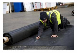
With an accurately measured, custom-cut, single-piece EPDM membrane, you know there are no vulnerable joins waiting to fail beneath the surface.
