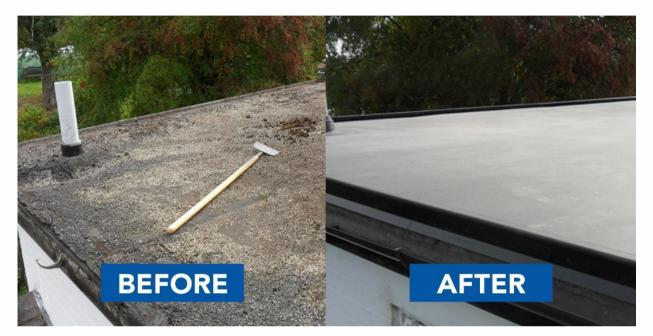
EPDM rubber sheet roofing has been around in the UK for a while, most commonly used in commercial flat roofing, modular buildings and façade waterproofing. In the last two decades, trade flat roofers have been bringing EPDM to the domestic market, due to the need for a sustainable replacement for traditional roofing materials.
