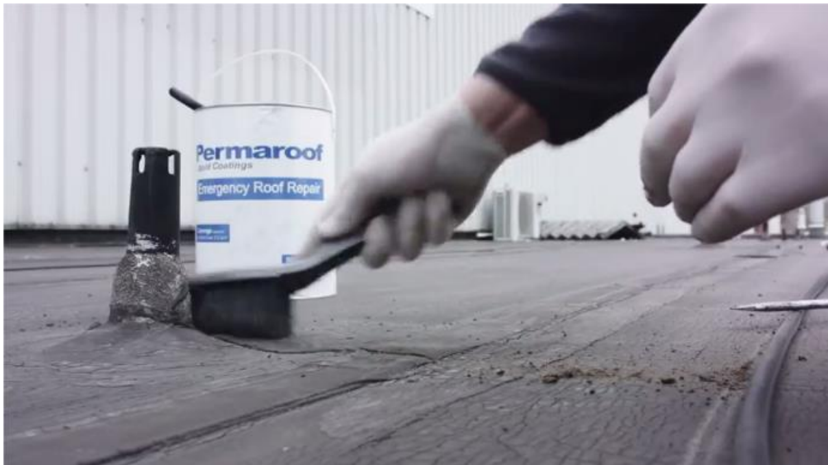
Fig 3 – Brushing away loose debris to complete preparation of the area.
