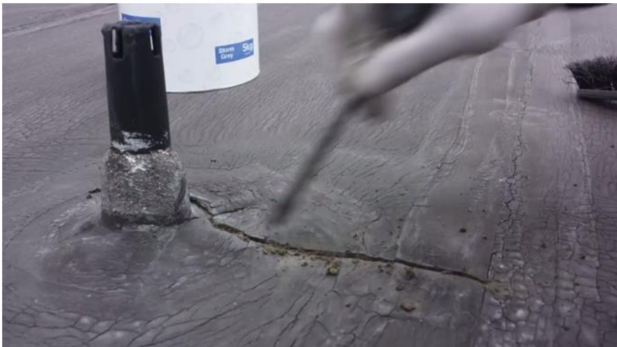
Fig 2 – Clearing the cracks of dirt and debris.
