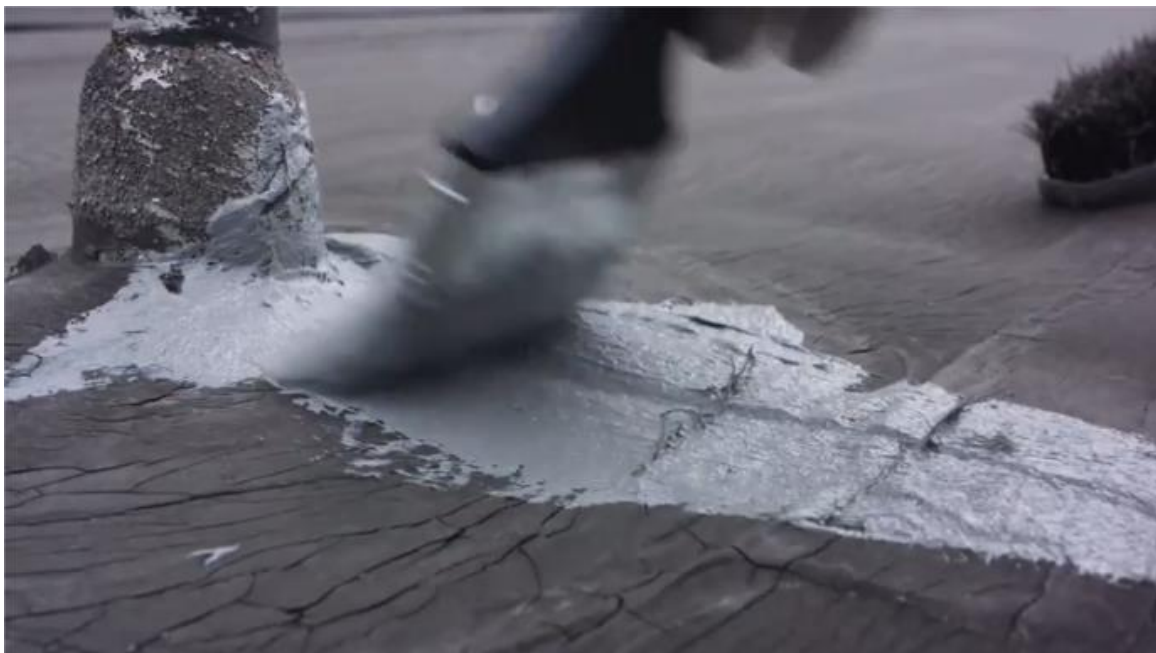
Fig 6 – Making sure the coverage is complete and even.
