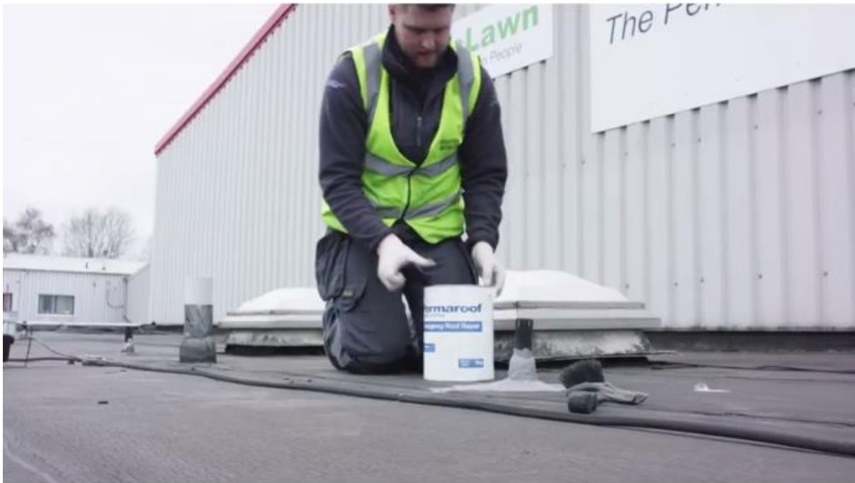
Fig 9 – Replacing the lid tightly.
