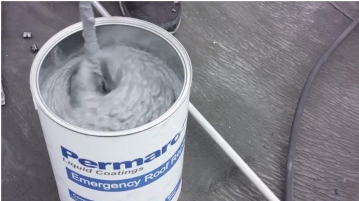
Fig 1 – Thoroughly mixing the Permaroof Emergency Roof Repair product.
